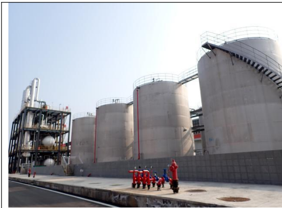
NMP 罐区围堰
